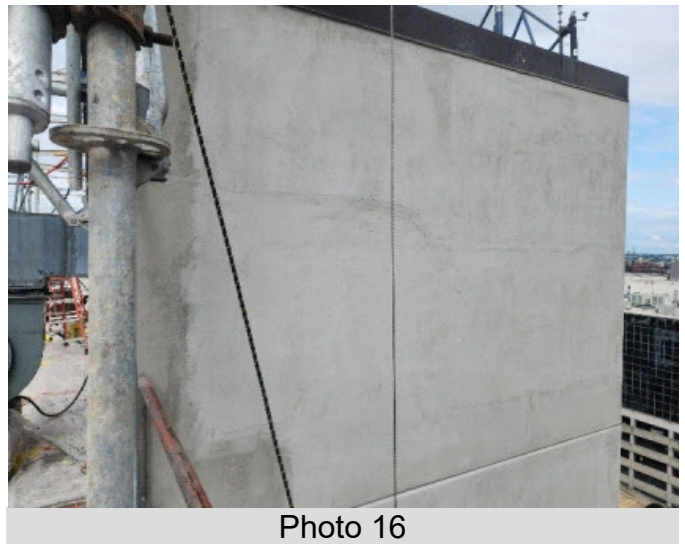
Wall surface after touch ups - no exposed mesh
